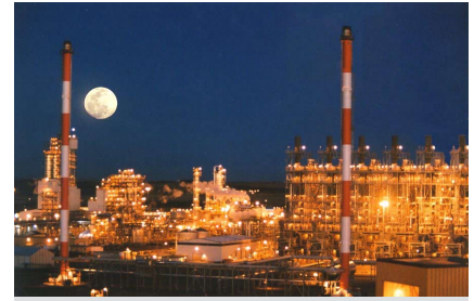
Nova Cracker Facility
