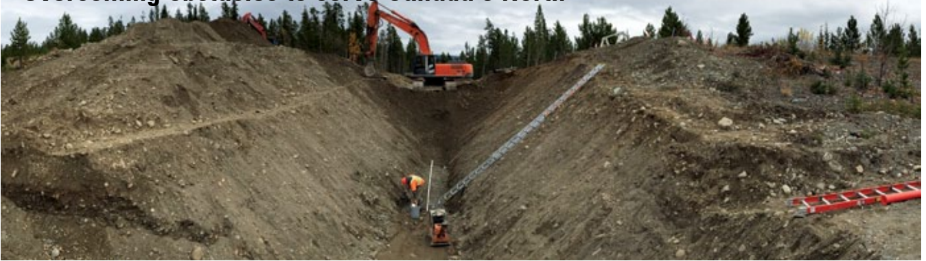
Hillcrest Water Main project. Photo courtesy of Castle Rock Enterprises.
