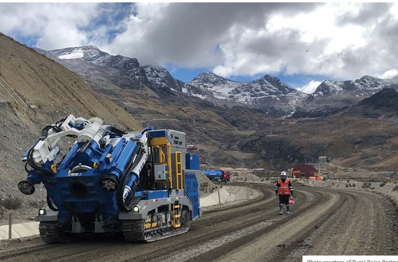
Photo courtesy of Tumi Raise Boring.
