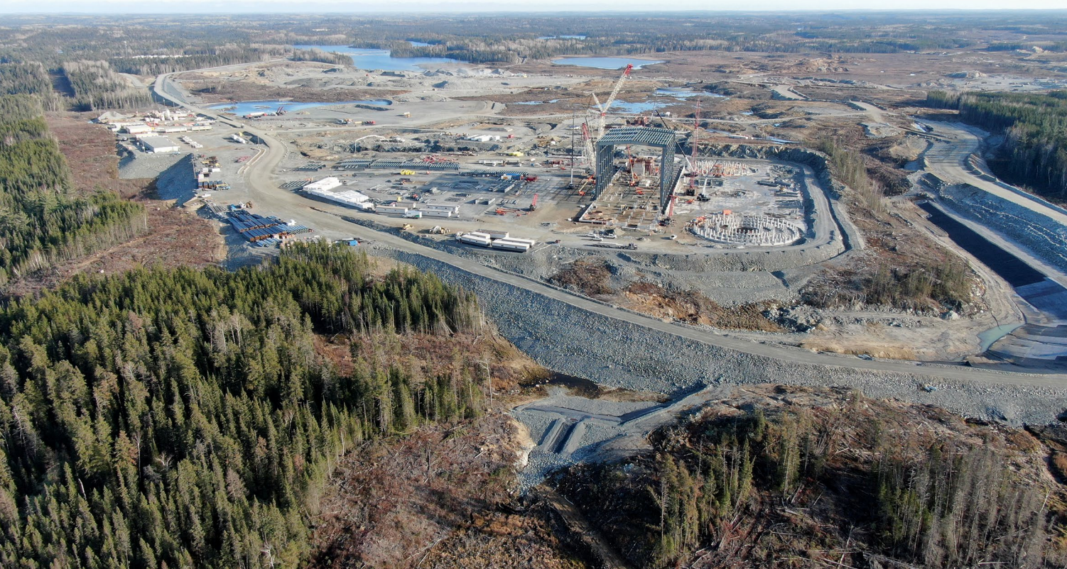
Côté Gold project. Image courtesy of IAMGOLD.
