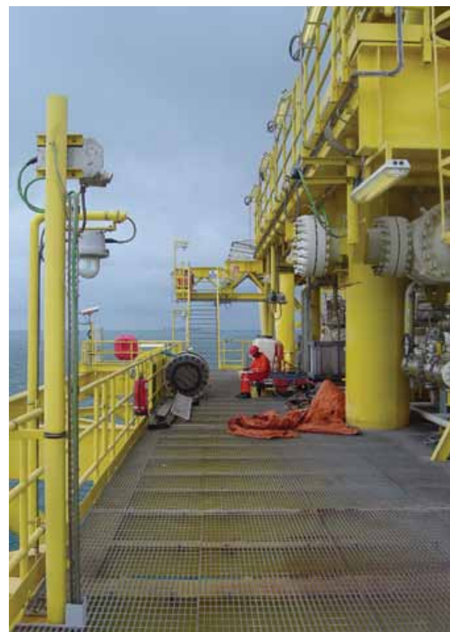
Offshore operations. Photo courtesy of Point Engineering.
