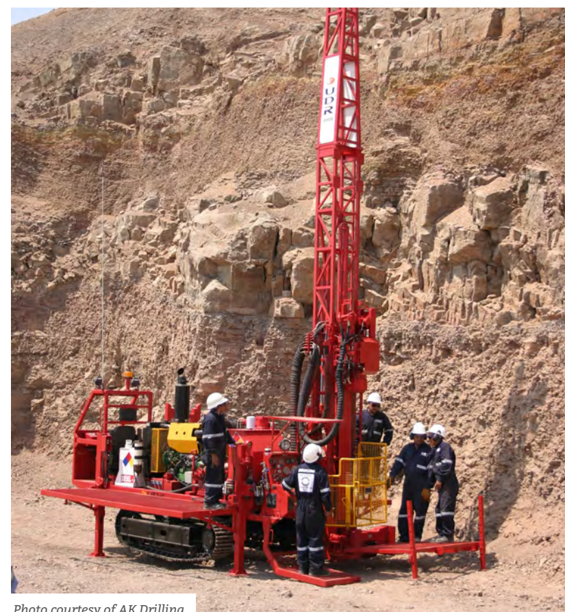
Photo courtesy of AK Drilling
