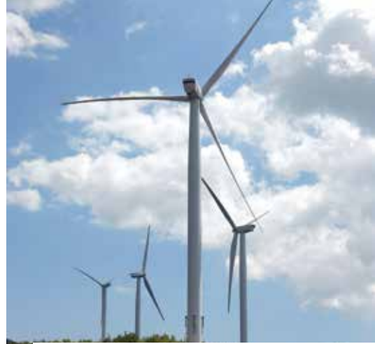
Wind farm. Zorlu Energy is currently constructing Turkey's largest wind farm in Osmaniye. Photo courtesy of Zorlu Energy.
