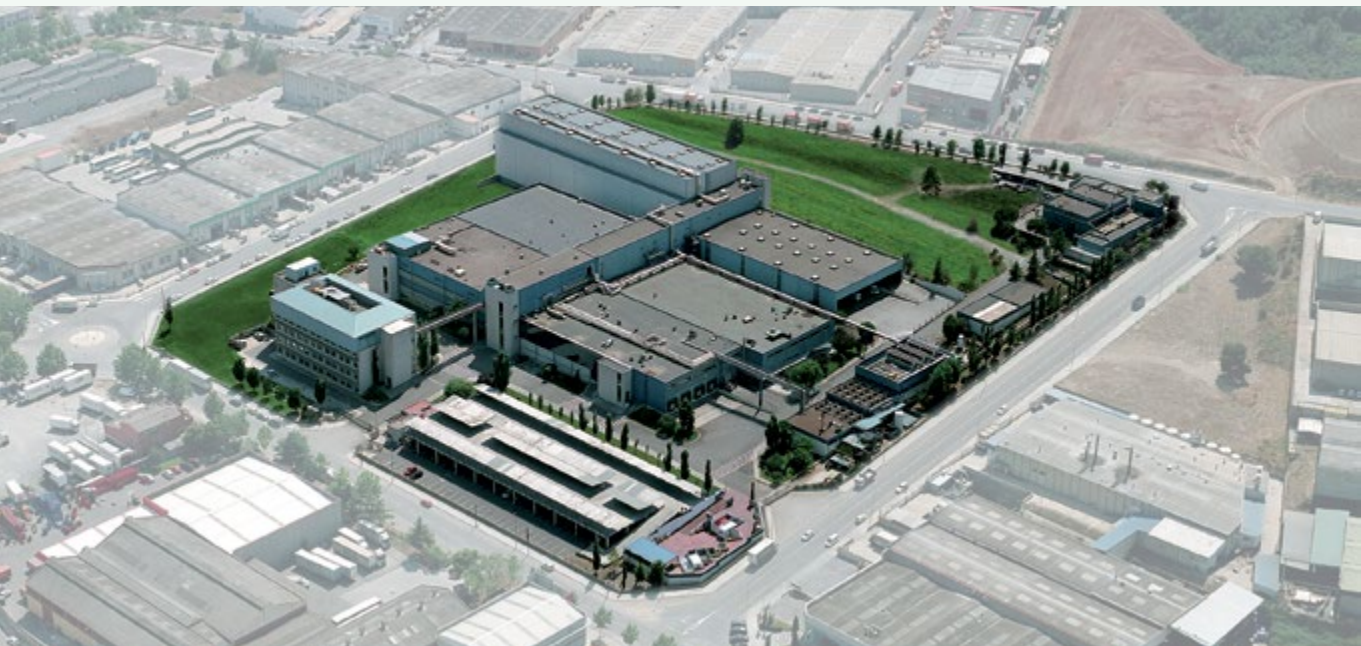
Image: Facilities for Kern Pharma pharmaceutical company in Terrassa (Barcelona)
