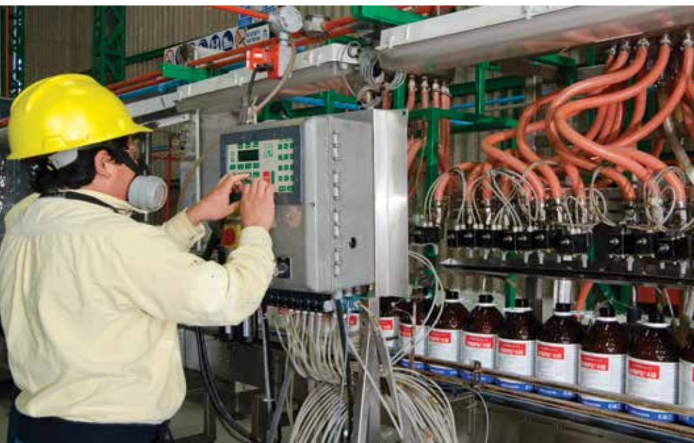
Chemical synthesis and blending manufacturing capabilities at Grupo Polak's Tlaxcala facilities. Photo courtesy of Grupo Polak.
