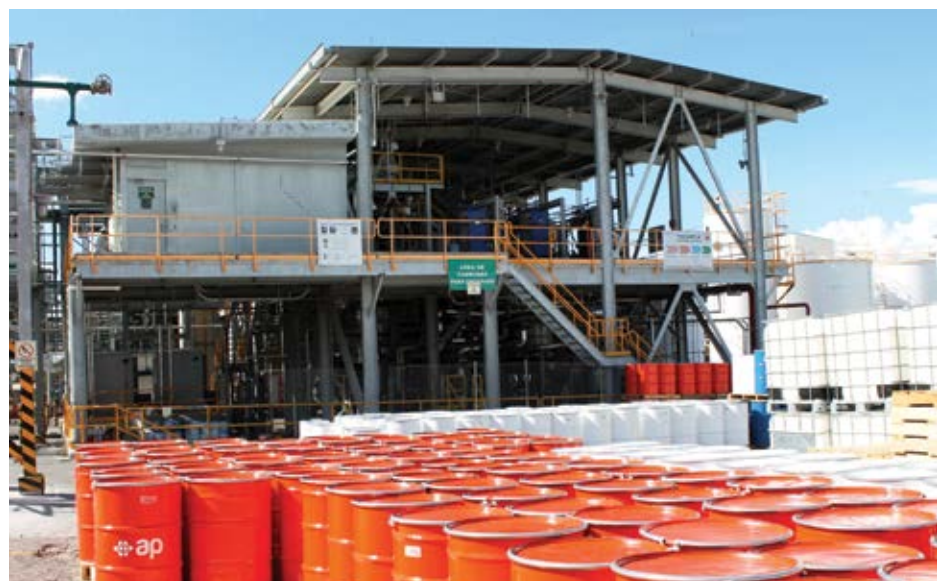
AP plant located in Queretaro, Mexico which develops high quality water and solvent based products. Photo courtesy of AP.
