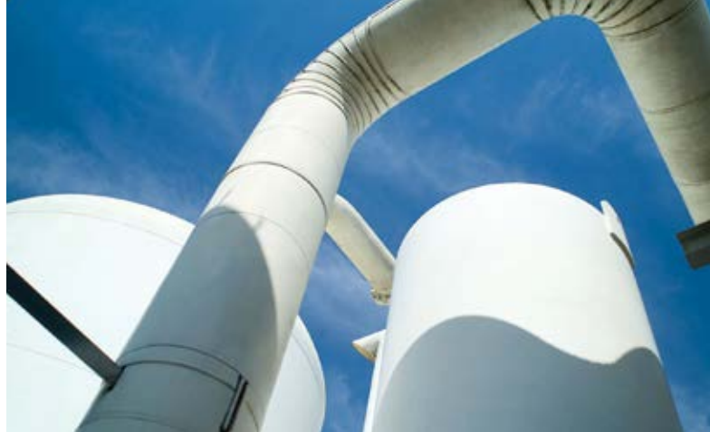
Inertization of ducts and pipes. Photo courtesy of Cryoinfra.
