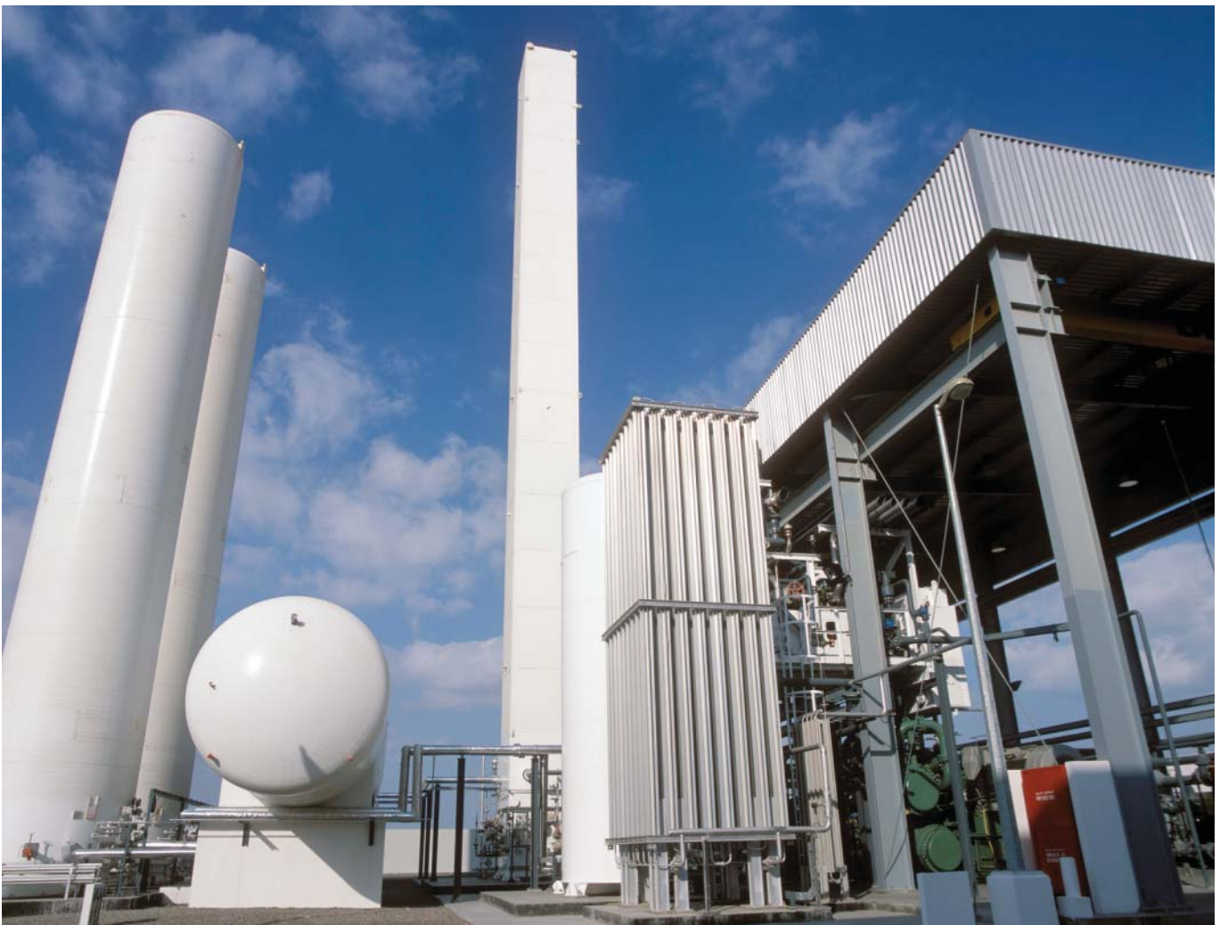
An Arabian Industrial Gases Co. plant in the UAE.
