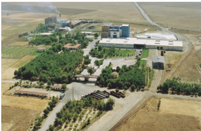
The Akkim Sodium Sulphate plant: Tapping the natural bounties.
