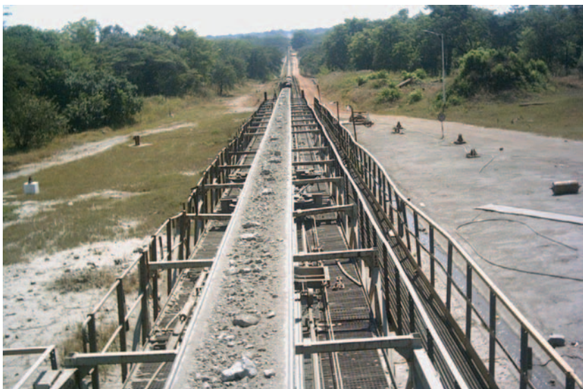
The Cable Belt Conveyor is the longest single drive conveyor in Africa. It has the unique feature of negotiating two horizontal curves. (Photo courtesy of Luanshya)
