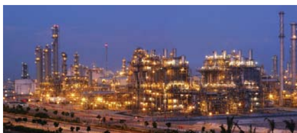
ExxonMobil Chemical's world-scale Singapore Chemical Plant has been operating on Jurong Island since 2001
