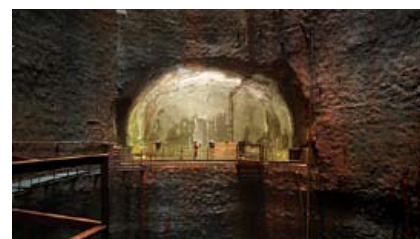
The Jurong Rock Cavern project will provide underground oil storage facilities
