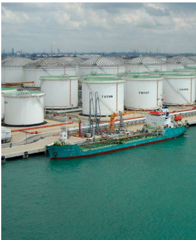
Rotary Engineering has worked on a range of recent storage projects, catering to growing regional distribution needs
