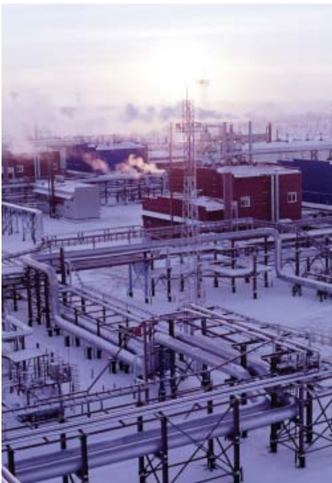
The Zapoliarnoye gas condensate field is one of the largest in the world. (Photo courtesy Sroytransgaz)
