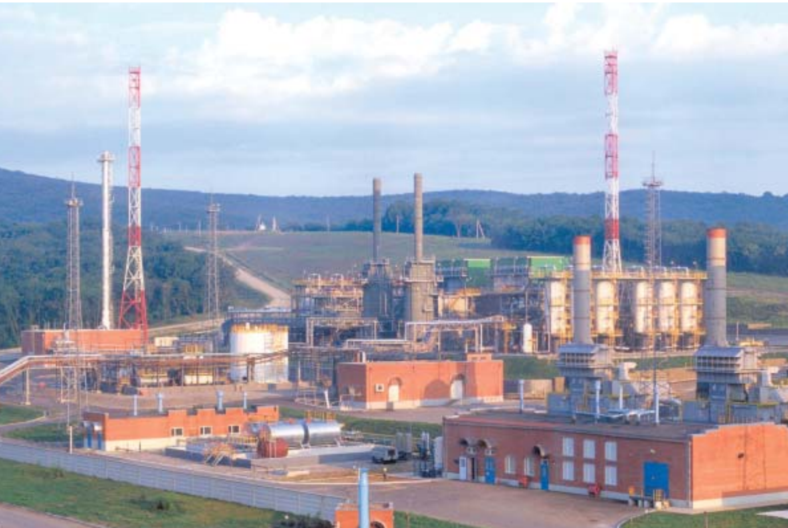
The Krasnodarskaya compressor station, part of the Blue Stream pipeline delivering Russian gas to Turkey. (Photo courtesy Stroytransgaz)
