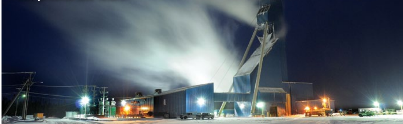
Casa Berardi, an old site shut down in the 1990s, was back into operation in 2006. (Photo courtesy of Aurizon Mines)
