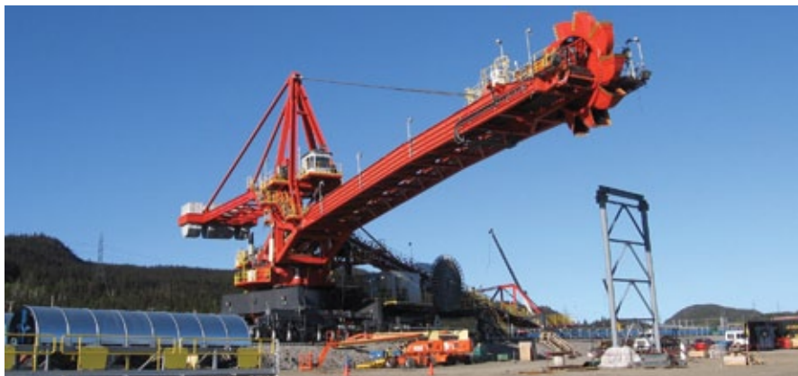
Pointe Noire stacker/reclaimer, operated by Cliffs. (Photo courtesy of CIMA+)
