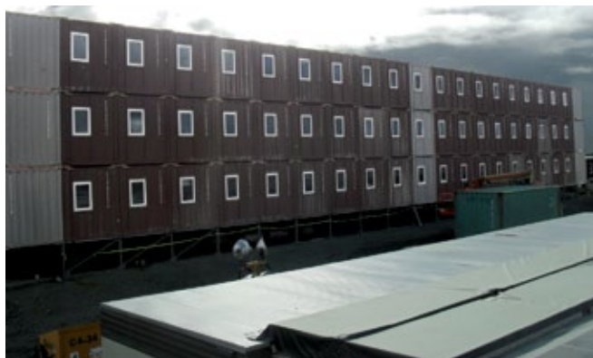
Tackling the lack of housing: modular homes at Canadian Royalties' Nunavik site. (Photo courtesy of Plugin Construction Solutions)
