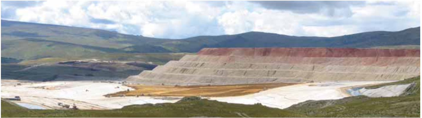
Buenaventura Ingenieros—geotechnical and civil works in gold mining unit, Cajamarca, Peru.
