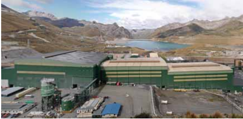
Concentrator plant located in Yanacancha that sits at more than 4,300 m above sea level. Antamina produces different mineral concentrates of which copper and zinc are the main products.
