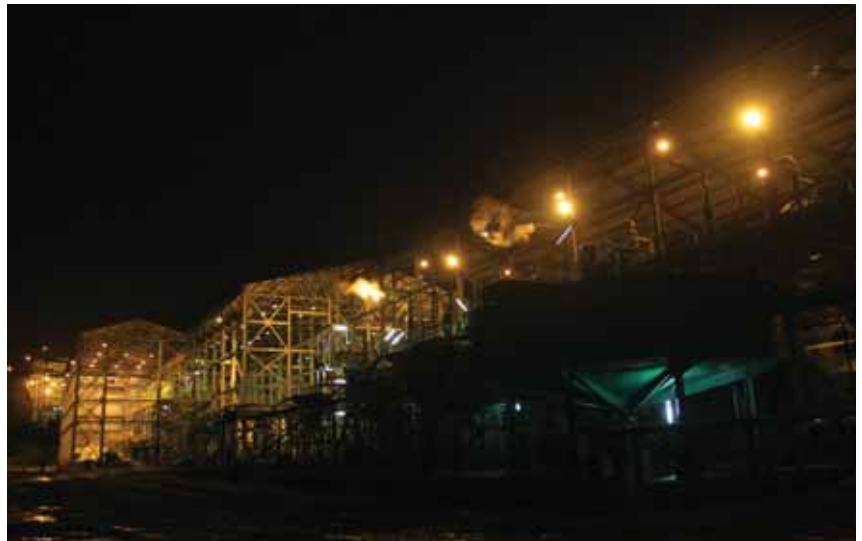
Cerro Lindo concentrator plant. The project is 100% owned by Milpo and is located 175 km in the south-east of Lima, in the Chincha province.
