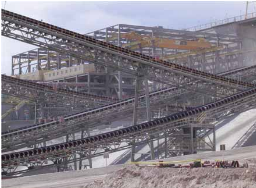
Buenaventura Ingenieros provided the concept for this crushing & grinding plant at a copper concentrator near Arequipa, Peru.
