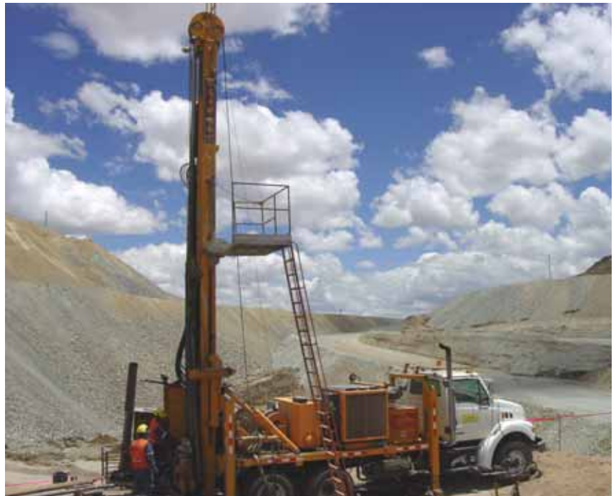
Geotec—Drilling at Tintaya mine.
