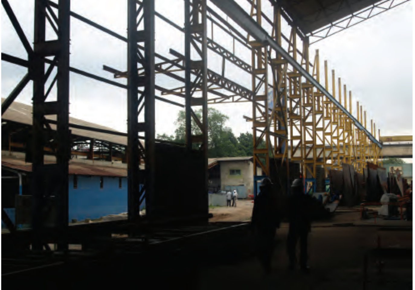
The Dorman Long fabrication yard in Lagos is a significant service provider.
