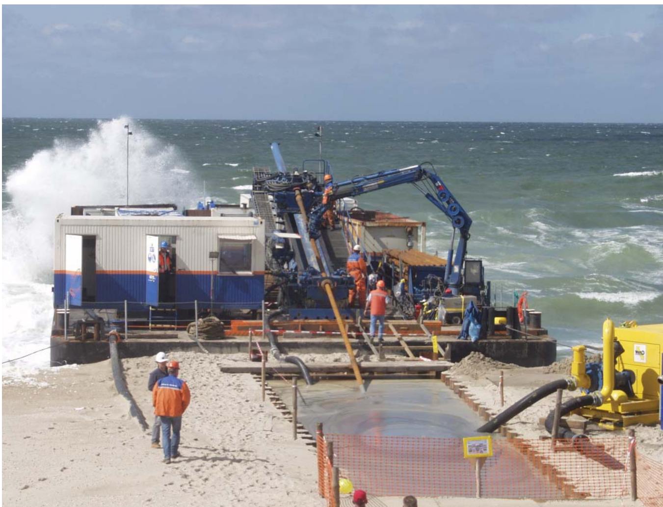
The BBL pipeline is being built between the Netherlands and the U.K. (Photo courtesy of Gasunie.)
