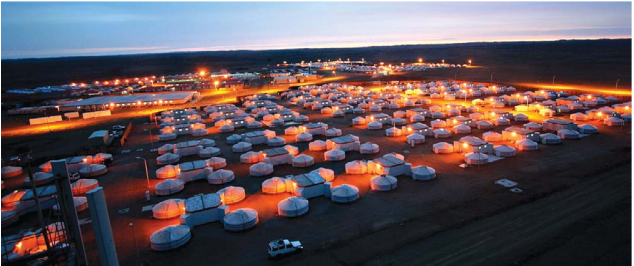
The main construction camp and administration center at Oyu Tolgoi (July 7, 2010).
