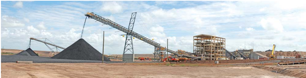
Energy Resources' coal handling and preparation plant, currently under construction in Mongolia, will be arranged similarly to what is shown here, but will be enclosed for protection against the elements. Annual plant capacity could reach 15 million mt.
