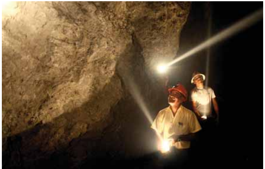
Underground works at El Sabinal, Ascencion, Northern State of Chihuahua.
