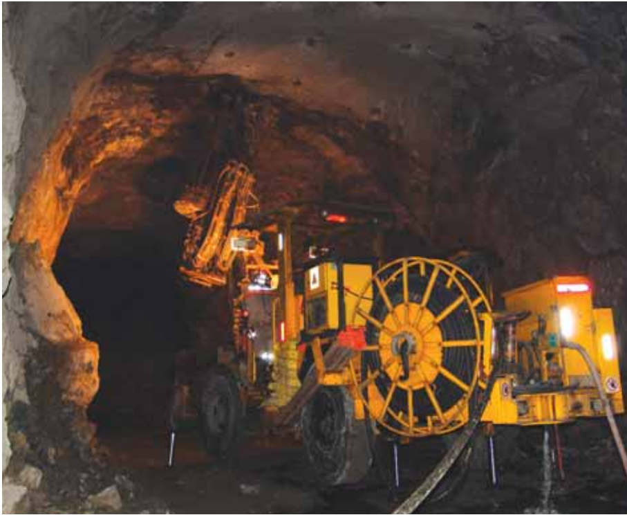
As more underground mines in Mexico prepare to increase production, equipment and technology will play a larger role. (Photo courtesy Atlas Copco)
