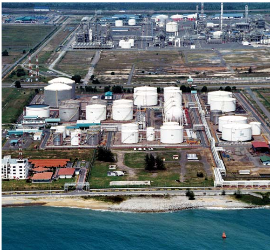
Kertih Terminals, operated in joint venture between Petronas, Vopak and Dialog Group, plays a key role on the complex’s logistical efficiency
