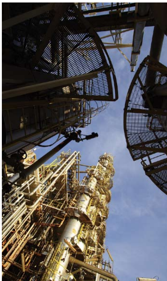
Petronas' Kertih Petrochemical Complex produces a rich array of petrochemical products
