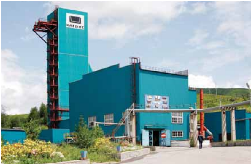
Head frame at Kazzinc Malevski mine. (Photo courtesy of Kazzinc)
