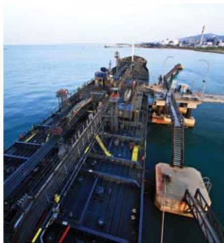
Bulk liquid chemical cargo discharging process at Polychemlindo's 20,000 DWT Jetty
