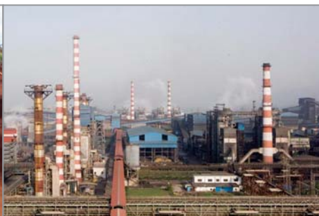
JSPL Steel Plant, Raigarh (Chhattisgarh), India
