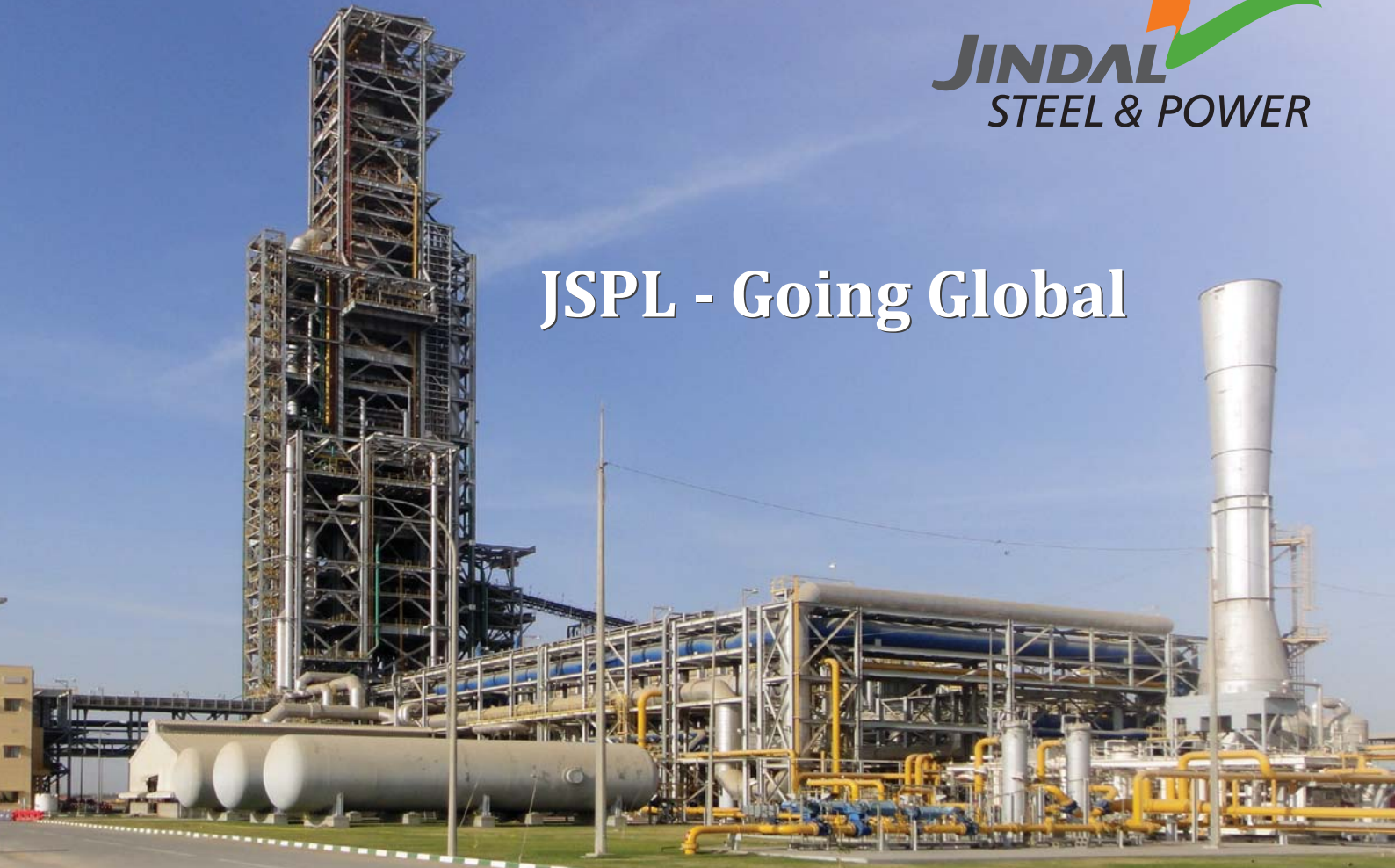
Jindal Shadeed Iron & Steel plant at Oman, Asia
