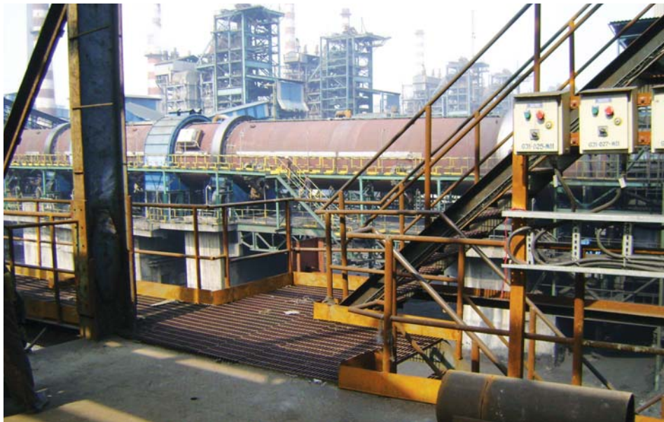
Bushan Steel is operating eight coal based DRI kilns melting the product in an EAF
