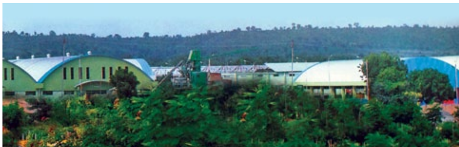
Technology at work: Supreme Industries' 131 acres plant at Gadegaon, Maharashtra.
