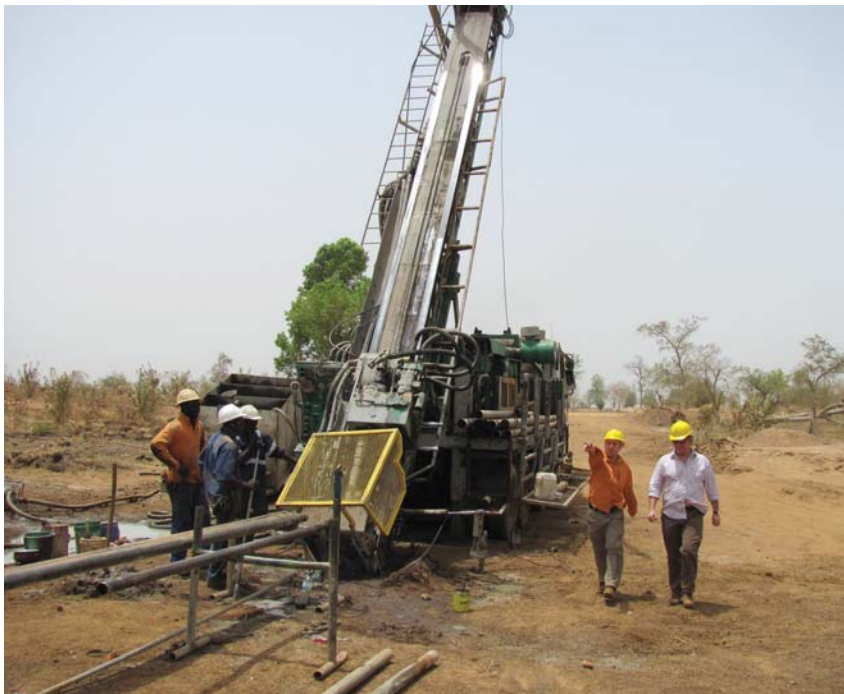
Core drilling at Kiaka. The Kiaka project lies at the intersection of the northeast striking Tenkodogo greenstone belt and the regionally significant north striking Markoye Fault, in whose proximity some of the larger gold resources discovered in Burkina Faso so far, have been discovered. These include lamgold's Essakane deposit (5.1 M oz), High River Gold's Taparko deposit (1.7 M oz), Orezone's Bombore deposit (2.1 M oz) and Etruscan's Youga deposit (1.5 M oz). (Photo Courtesy of Volta Resources)
