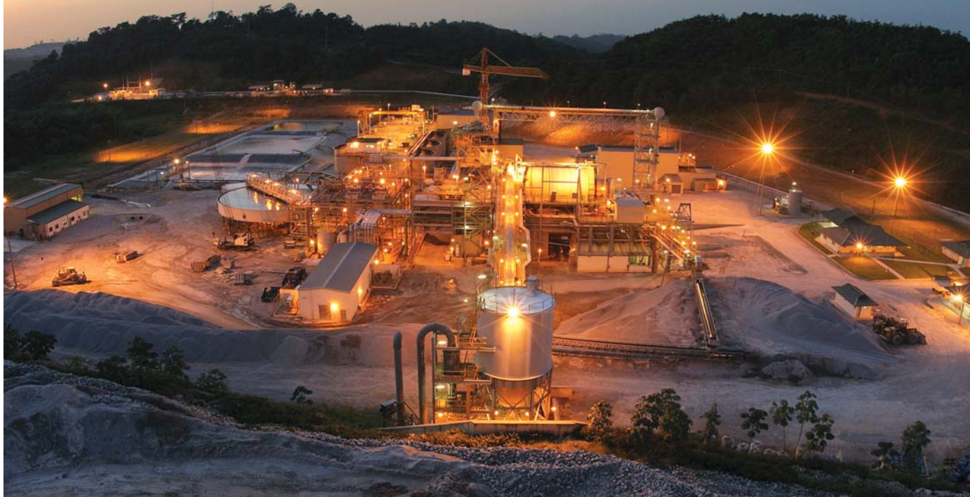
Gold Fields Tarkwa mine, located in southwestern Ghana, recently completed the construction of a CIL plant that is expected to increase throughput to 1 million tons of ore per month on a sustainable basis. (Photo courtesy of Gold Fields Ghana Ltd.)
