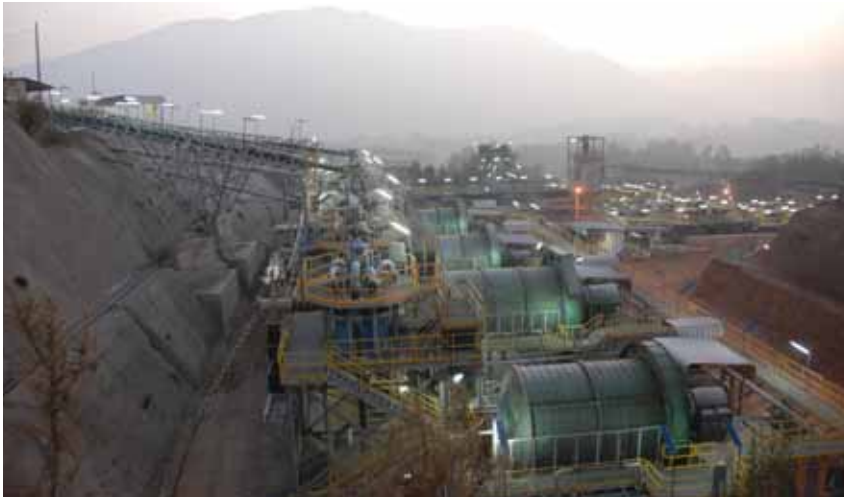
Minera Valle Central produces copper and molybdenum concentrates from the tailings of Codelco's El Teniente mine. (Photo courtesy of Rory Sheldon)
