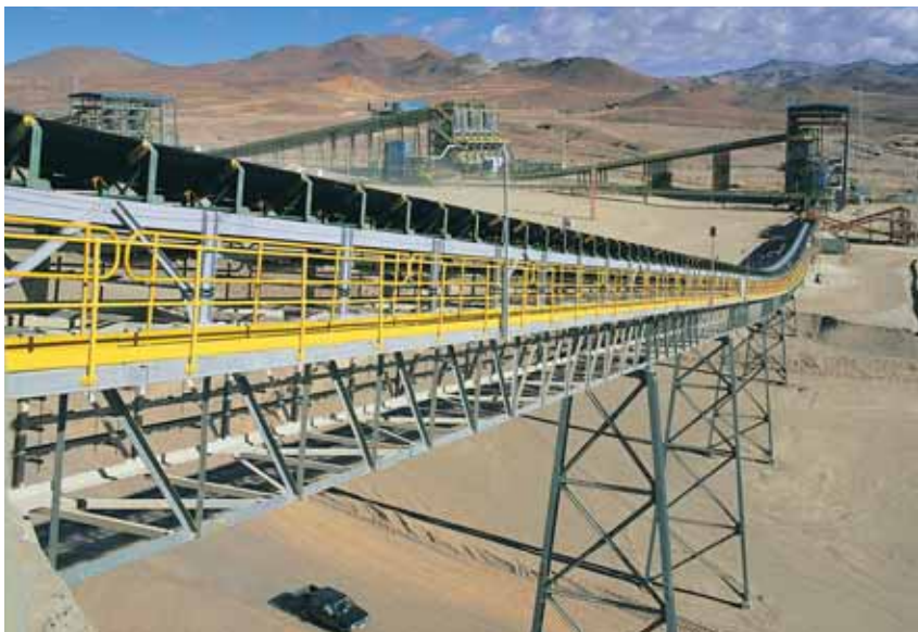
The conveyor galleries at El Abra are a prime example of the engineering required by modern mining operations.
