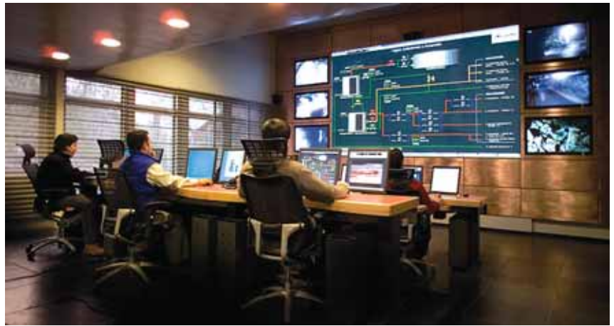
Chilean copper miners employ state-of-the-art technology, such as the Andina control center, to keep their competitive edge. (Photo courtesy of ABB)
