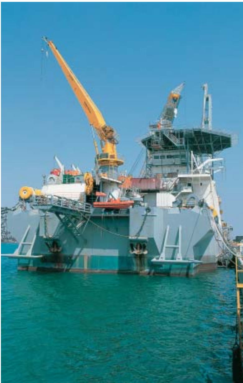
Operations in the Caspian benefit from the introduction of some of the latest engineering technology. Shown here is Israfil Husseyinov , McDermott's pipe-laying barge.
