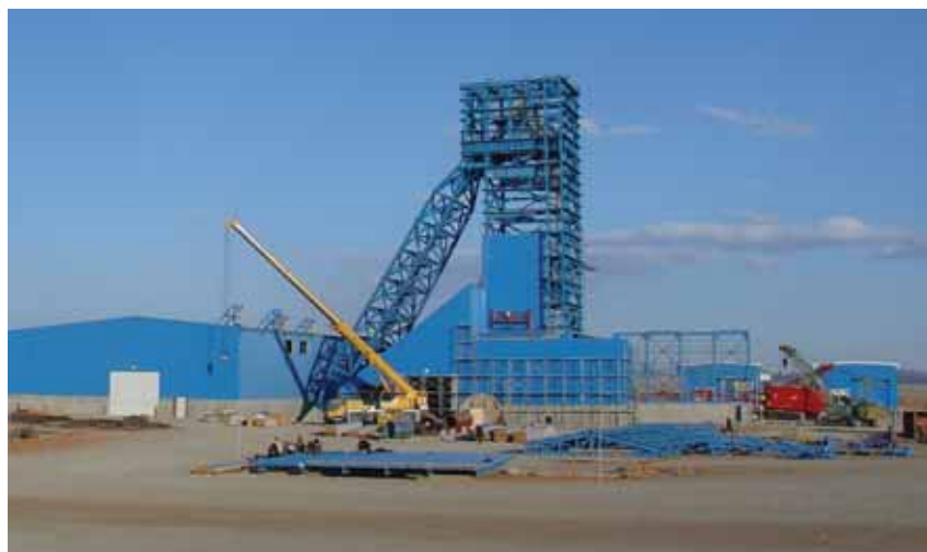
Construction of the headframe and surface plant for Ivanhoe Mines' Oyu Tolgoi project in Mongolia. According to JS Redpath President and CEO George Flumerfelt, "Bearing the Canadian flag doesn't guarantee us success [in business], performance does." (Photo: JS Redpath Group)
