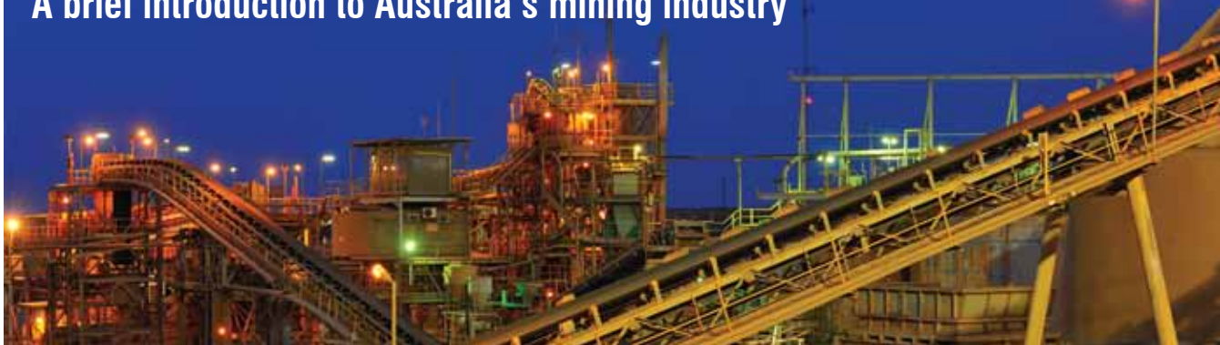
Conveyors at Newmont Boddington Gold Mine (photo courtesy of Newmont)
