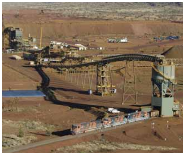
Train loading at BHP Billiton's iron ore operations at Mine Area C in the Pilbara.
