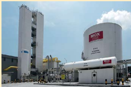
Mox-Linde (Linde Group's Malaysian subsidiary) air separation plant in Pasir Gudang, Johor
