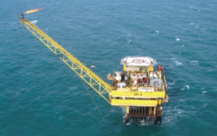
Mechanical mounting and instrumentation on an offshore platform in the Magellan Strait. (Photo courtesy EDVSA)
