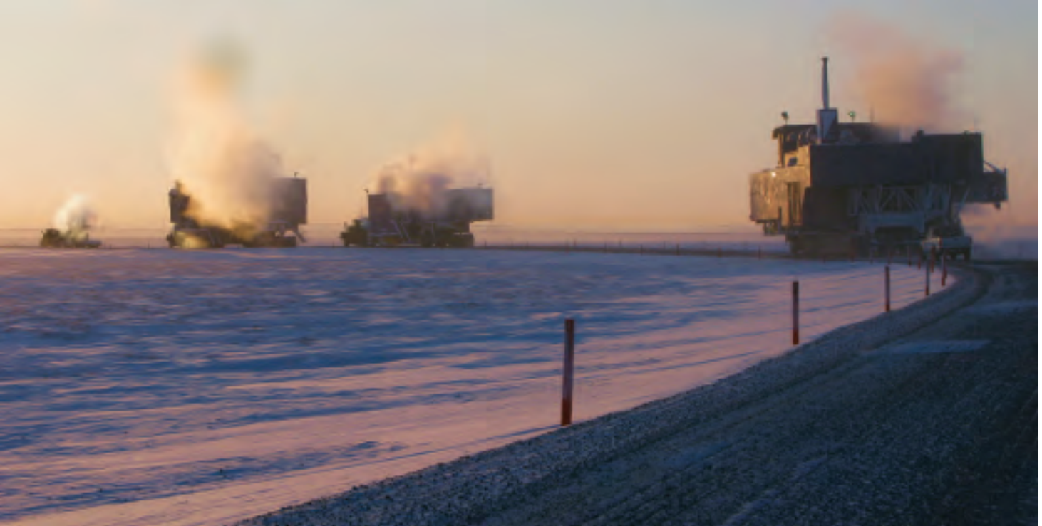
Drilling season on the North Slope takes place in the winter, from December to April. Snow and ice build-up allows for easier transport of heavy equipment across the tundra surface.
