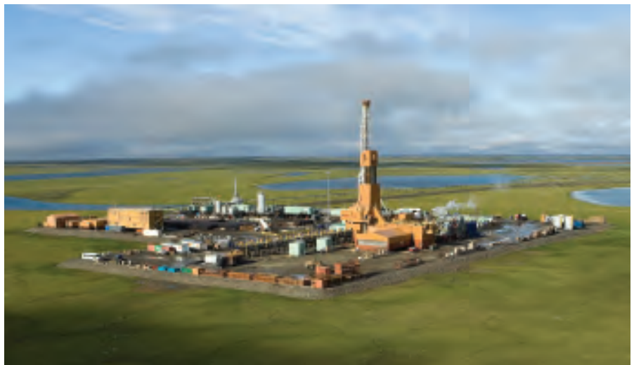
Alpine satellite CD-2 is connected to the main Alpine pad by a combination gravel road/airstrip.
