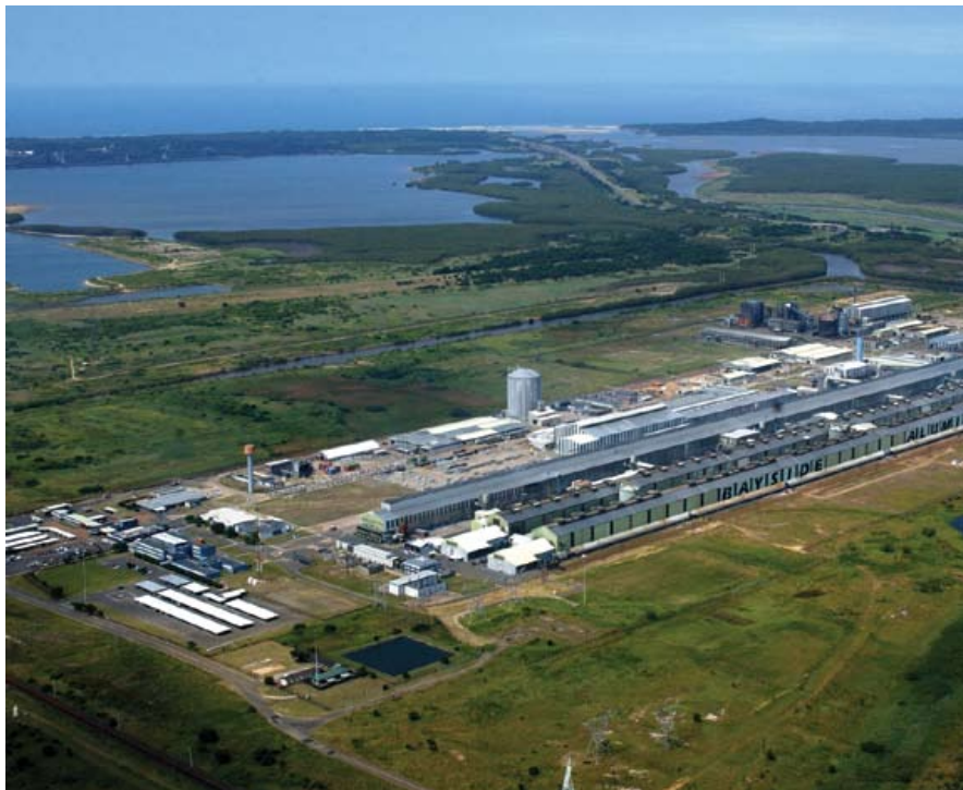
Aluminium smelter in Richards Bay. (Photo courtesy of BHP Billiton)
