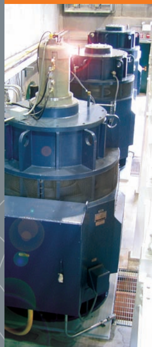
1.5 MW Hydrogenerators 4,400 volts, 60 Hz, 16 pole, 450 RPM
