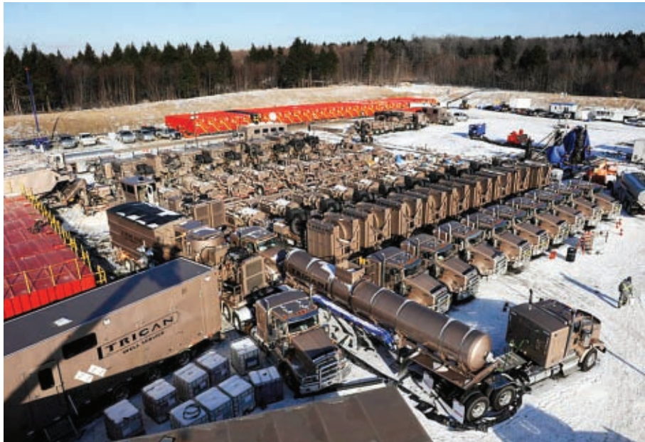
Trican's equipment at a fracturing operation in the U.S. Marcellus shale.
