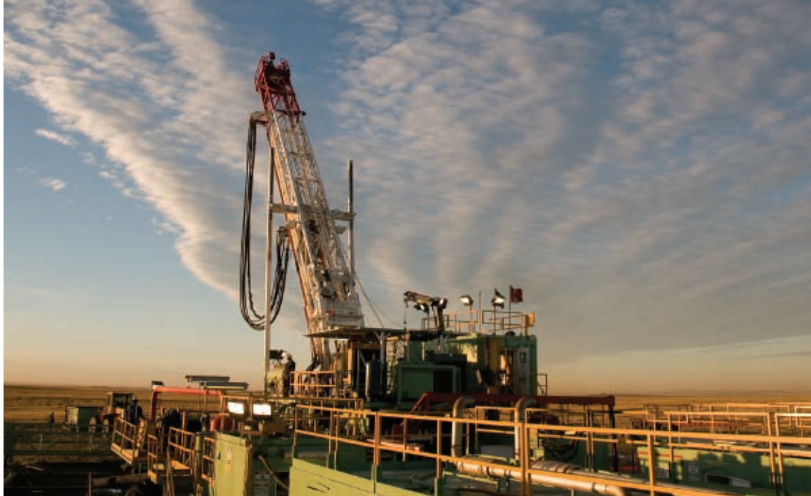
A super single rig designed and built by Precision Drilling, operating 100 kilometers northeast of Calgary in Rosebud, Alberta, for Encana.
