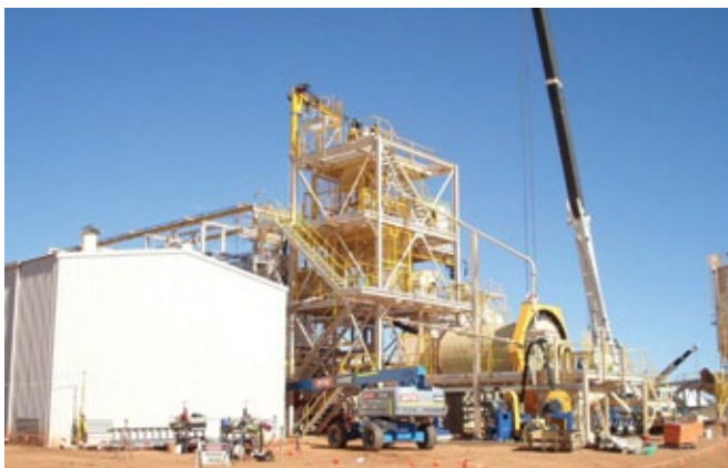
Installation of the ball mill. Photo courtesy of Doray Minerals.
