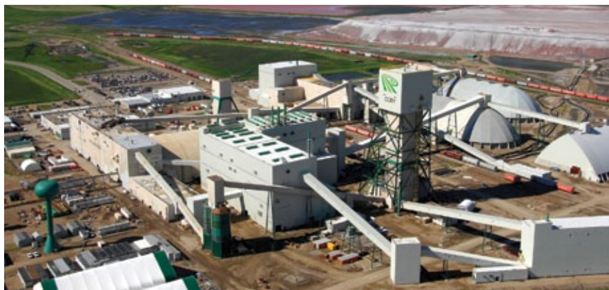
Graham has successfully completed numerous projects at PCS' Cory facility.
