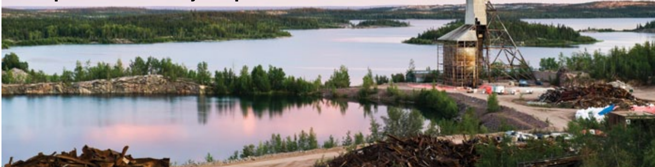
View of the Gunnar Mine site during summer 2011. The buildings and headframe have since been removed due to safety concerns. Photo courtesy of the Saskatchewan Research Council (SRC).
