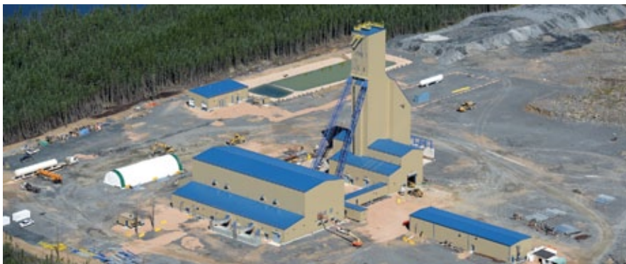
The hoisting system in the main ventilation shaft at Hudbay's Lalor project is now capable of hoisting 1,400 mt of combined ore and waste per day, with completion of the production shaft and new concentrator expected in late 2014. Photo courtesy of Hudbay.
