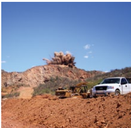
First blast. (Photo courtesy of SilverCrest).
