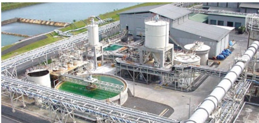
PT Smelting's waste water treatment plant. Photo courtesy of PT Smelting.
