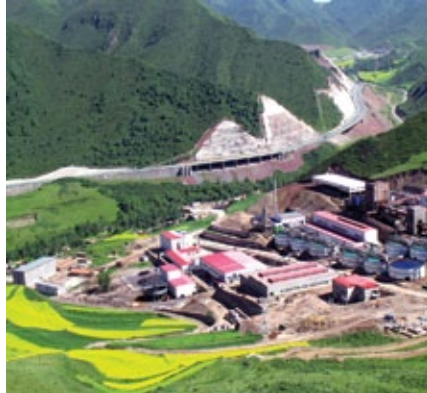
Reduction roasting and ammonia leaching plant. Photo courtesy of BGRIMM.
