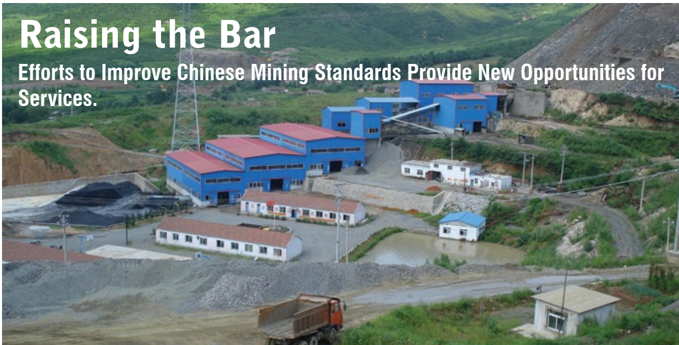
Hanking's Mengjia iron ore processing plant located in Benxi, Liaoning province. Photo Courtesy of SRK Consulting.
