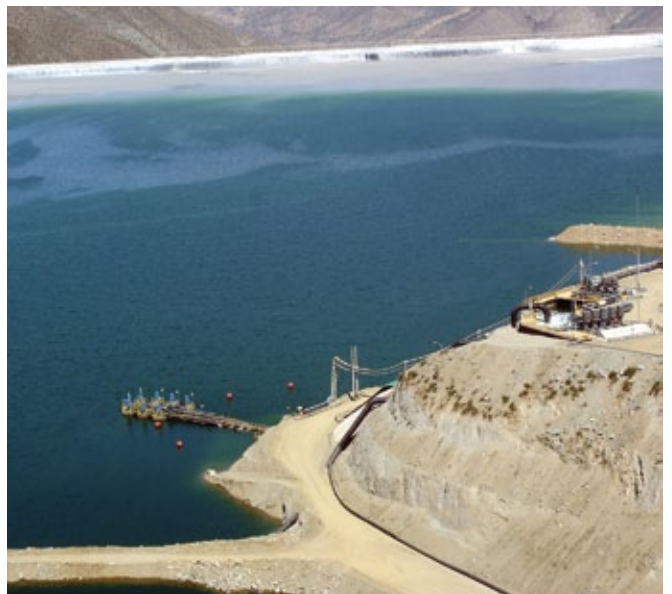
Tailing dam engineered by JRI Ingenieria. (Photo courtesy of JRI).
