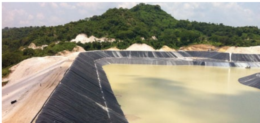
A waterlogged site in Nicaragua, Photo Courtesy of Esinsa
