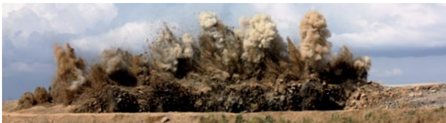
Rock blasting. Photo courtesy of Austin Powder.
