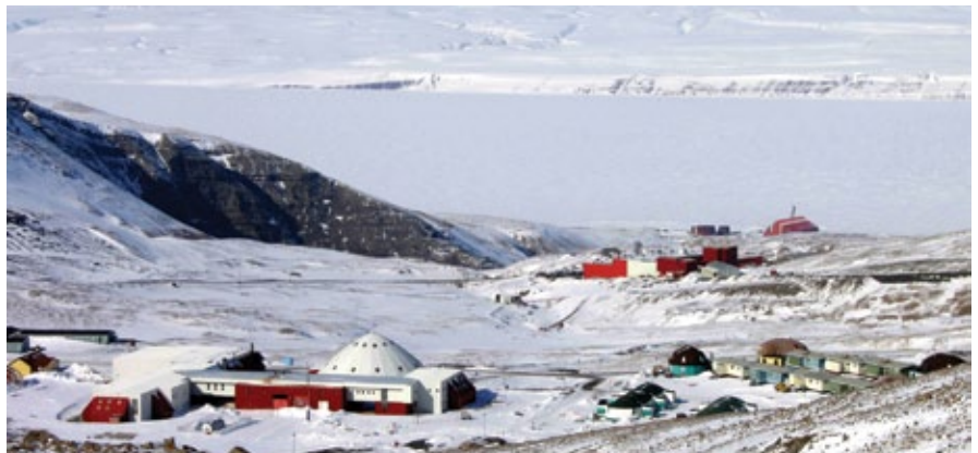
Nanisivik mine remediation, Nunavut. Photo courtesy of AECOM.
