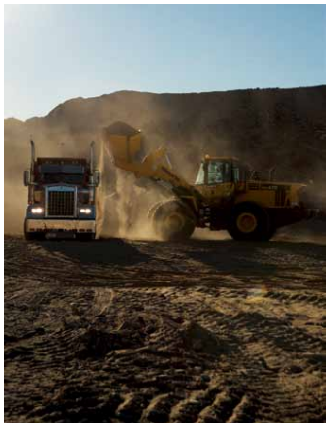
Earthmoving activities at Baja Mining's Boleo site
