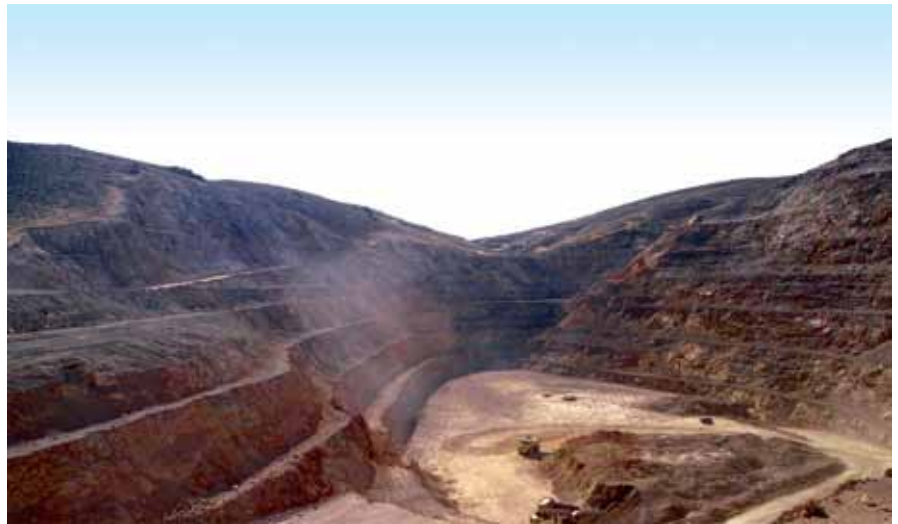
Ausenco provided innovative heap leach and run-of-mine design services to the technically demanding Lomas Bayas, an open-pit copper mine located in the Atacama Desert, Chile.
