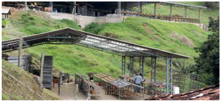
Over 30,000 metres of drill core is stored at Sunward Resources' new core shacks at the Titiribi project, Antioquia, Colombia.
