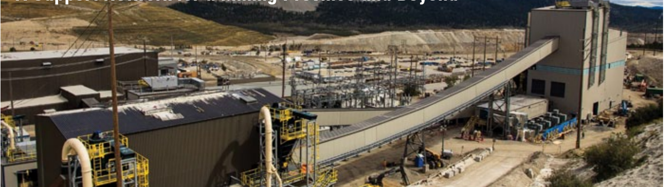
Pebble crusher at Highland Valley Copper Mill project in British Columbia (Owner: Teck Highland Valley Copper Partnership). Photo courtesy of Fluor.
