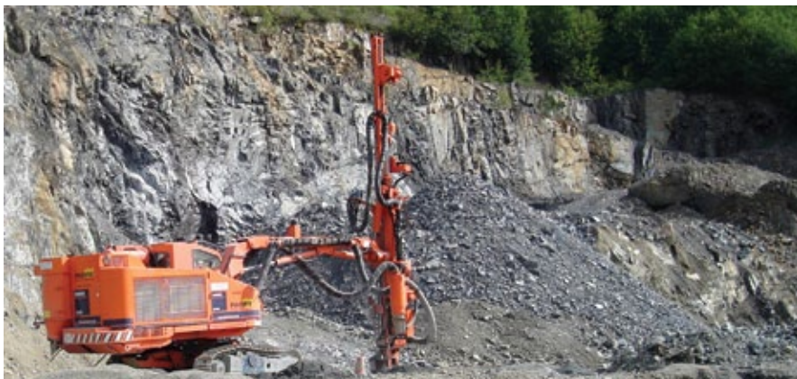
Drilling operation. Photo courtesy of Pacific Blasting and Demolition.
