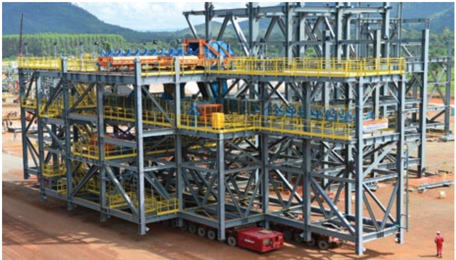
Mammoet's first module for Vale's S11D. Photo courtesy of Mammoet.
