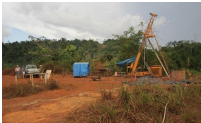
Belo Sun launched a large diamond drill program to upgrade and expand their Volta Grande project, preparing it for a definite feasibility study in Q1 of 2013. Photo Courtesy of Belo Sun.
